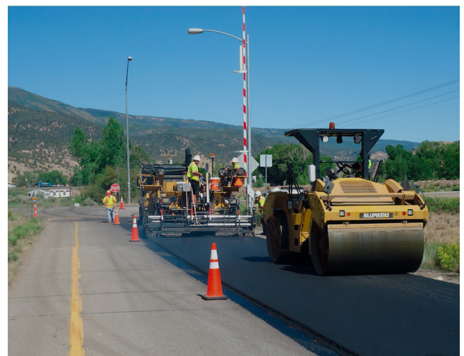
Crew works on repaving and other safety improvements Source: CDOT
