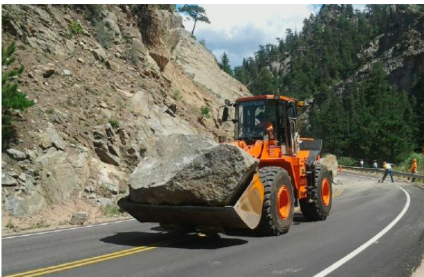
Crew removed rock debris on State Highway 119 Source: CDOT, 2020
