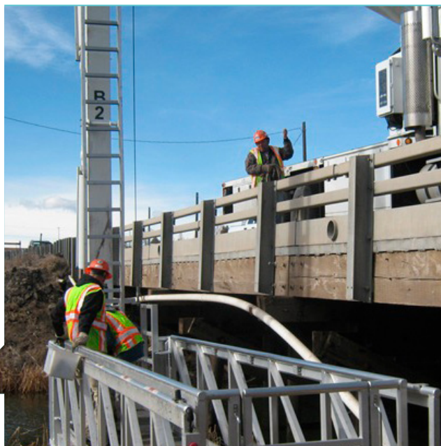
Crew works on bridge repairs. Source: CDOT, 2020
