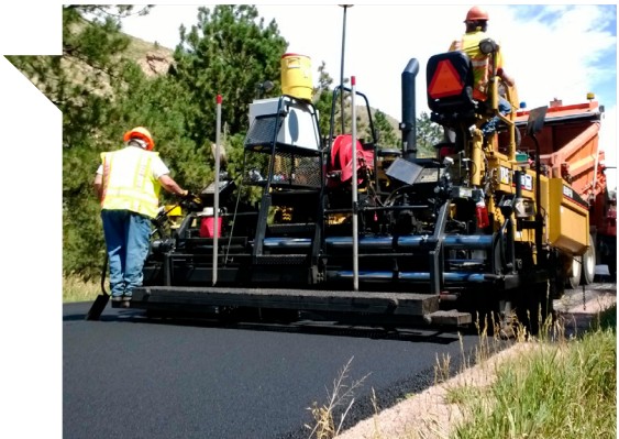
Crew working on rural paving Source: CDOT, 2020
