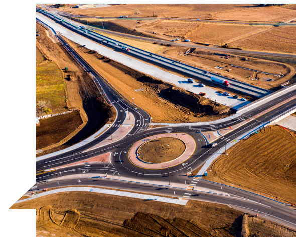
Construction on Interstate 25 Source: CDOT, 2020
