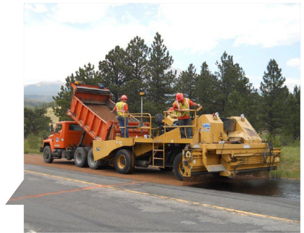
Crew works on State Highway 7 Source: CDOT, 2020
