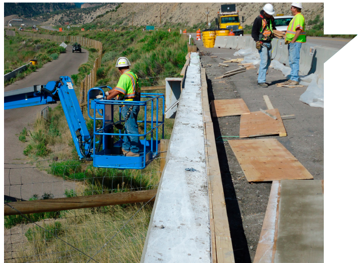
Crew working at guardrail construction site Source: CDOT, 2020
