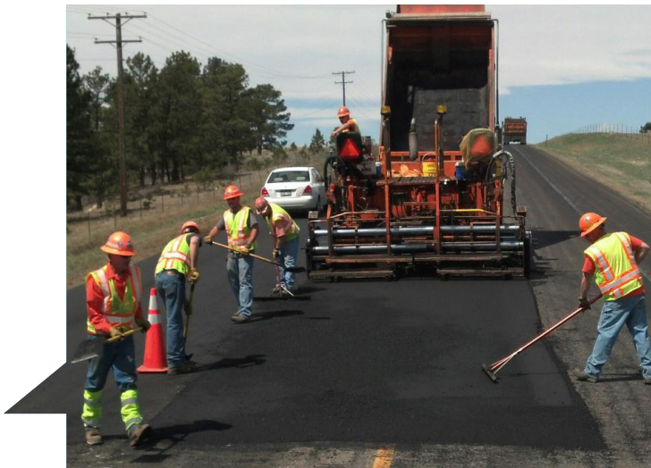
Crew works on rural paving along State Highway 86 Source: CDOT, 2020
