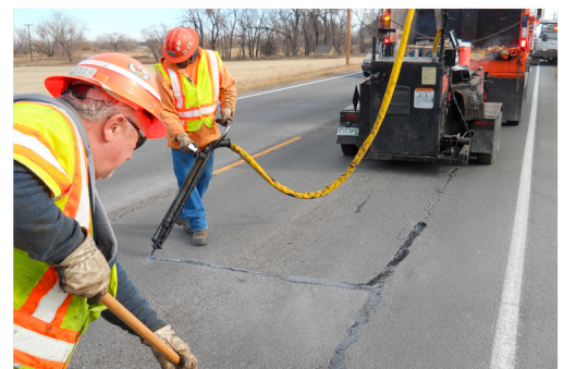
Crew seals cracks on Highway 7 Source: CDOT, 2020
