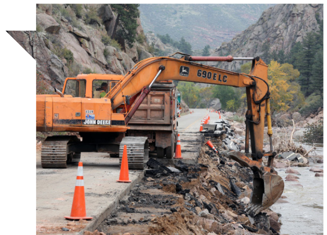
Crew begins repairs after 2013 flooding event Source: CDOT, 2020
