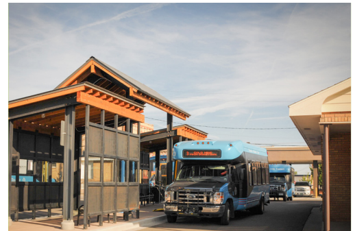
Buses arrive at all points transfer center Source: FHU, 2020
